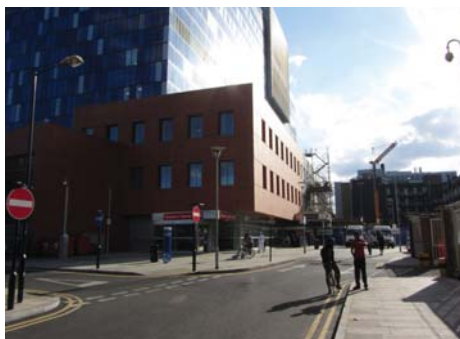
Current view from Raven Row looking west towards new Royal London Hospital entrance
