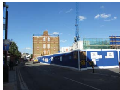
Current view from east along Durward Street
